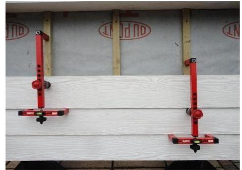
When the soffit is reached the last full width board will require the Cladman roller to be repositioned. Referring to the UNDER SOFFIT OVERLAP GUIDE, move the roller to the position recommended for the board width. Mark the overlap distance on the last board, align the top of the roller with the mark and fix to the baton.
