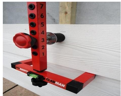
We recommend using the 8mm driver bit supplied in a battery drill to screw the Cladman to a baton (at least one in from the end of the board). Repeat the procedure fitting another of the Cladman at the other end of the board.
