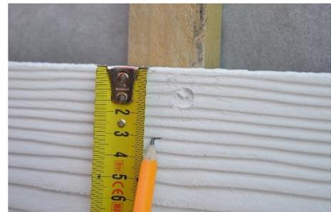
With the lower legs positioned firmly under the lower edge of the board, observe if the top of the roller aligns with the overlap mark. If adjustment is required simply slacken the locking knob and rotate the lower legs until alignment is achieved, retighten the locking knob. Now the Cladman is now set and all overlaps will be the same.
